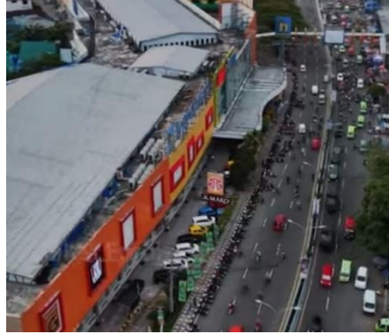
Figure 9. Alternative Condition 5 Source: Observation Results, 2024
