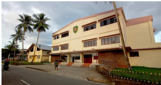
Figure 7. Alternative Condition 3 Source: Observation Results, 2024
